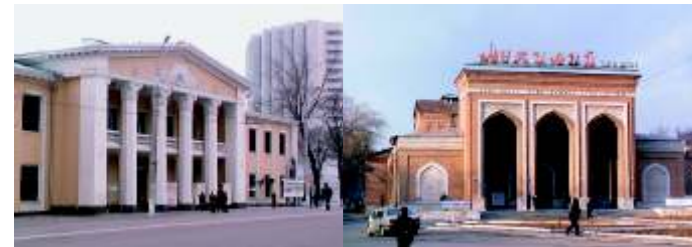
Installations: Central Concert Hall Officer of Military of Russia Moscow, Mukimi Theater Tashkent
